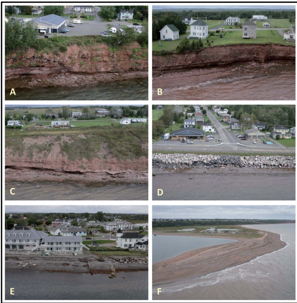
Figure 11. Examples of exposed features in different coastal settings: (A) commercial building – rock cliff; (B) primary residences – rock cliff; (C) railway – unconsolidated cliff with rock base; (D) provincial highway, aqueduct and sewer system, and stores – low unconsolidated cliff with rock armour; (E) commercial buildings (motel) – beach terrace; and (F) warehouse, campground facilities and aqueduct – spit.
